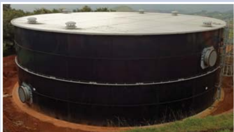
Trough Deck Roof
