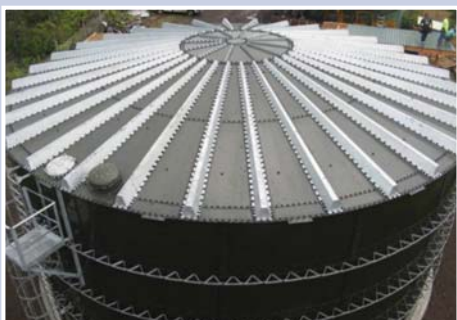
Glass-Fused-to-Steel Roof
